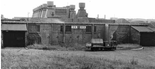
The exit end of the rolling house (Building 809) in the 1940s
